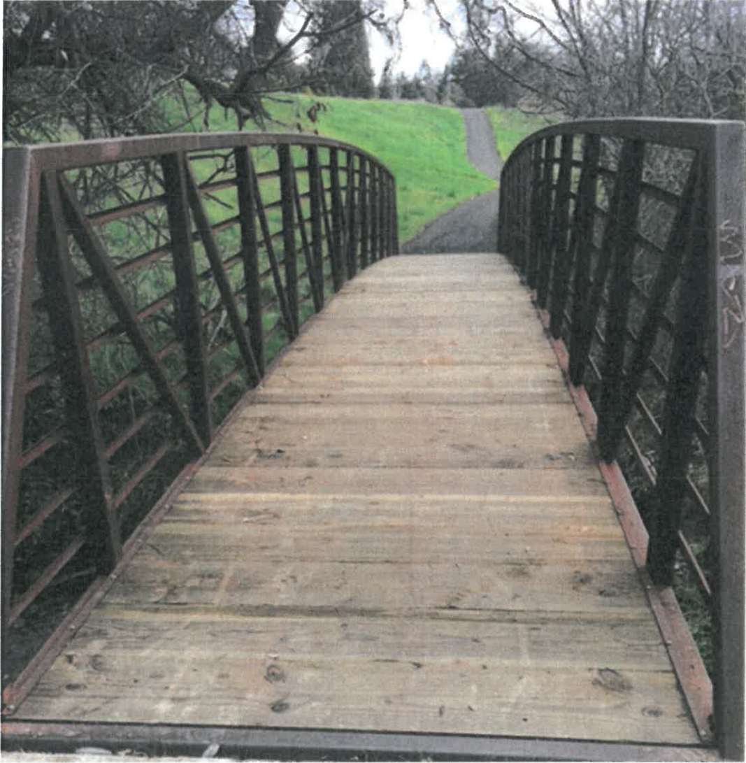
After replacement of wood deck
